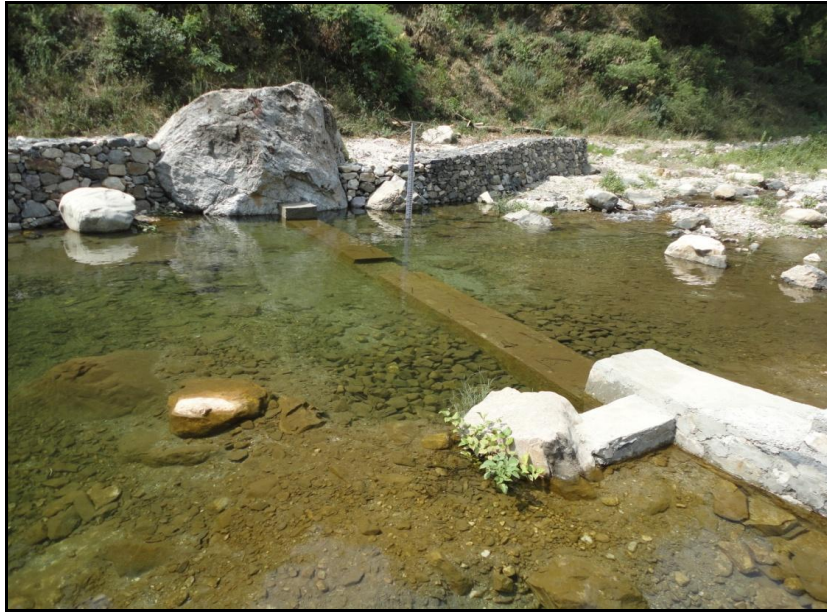
Fig. 3. 2 Discharge weir at Jijali
