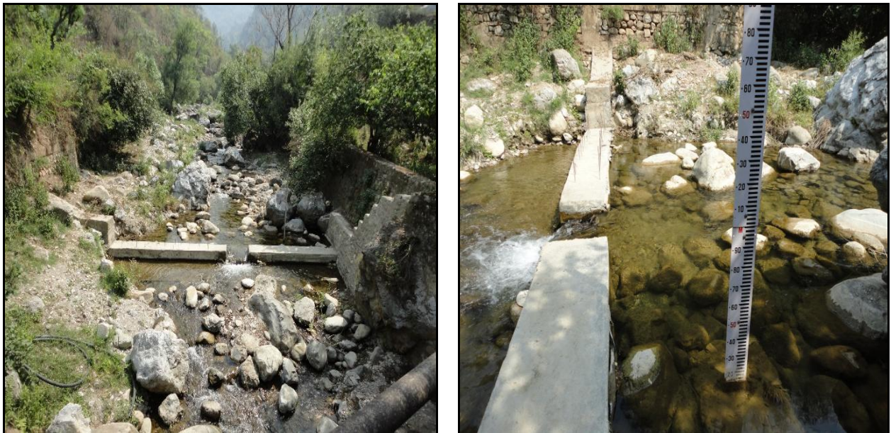
Fig. 3. 1 Discharge weir at Herval
